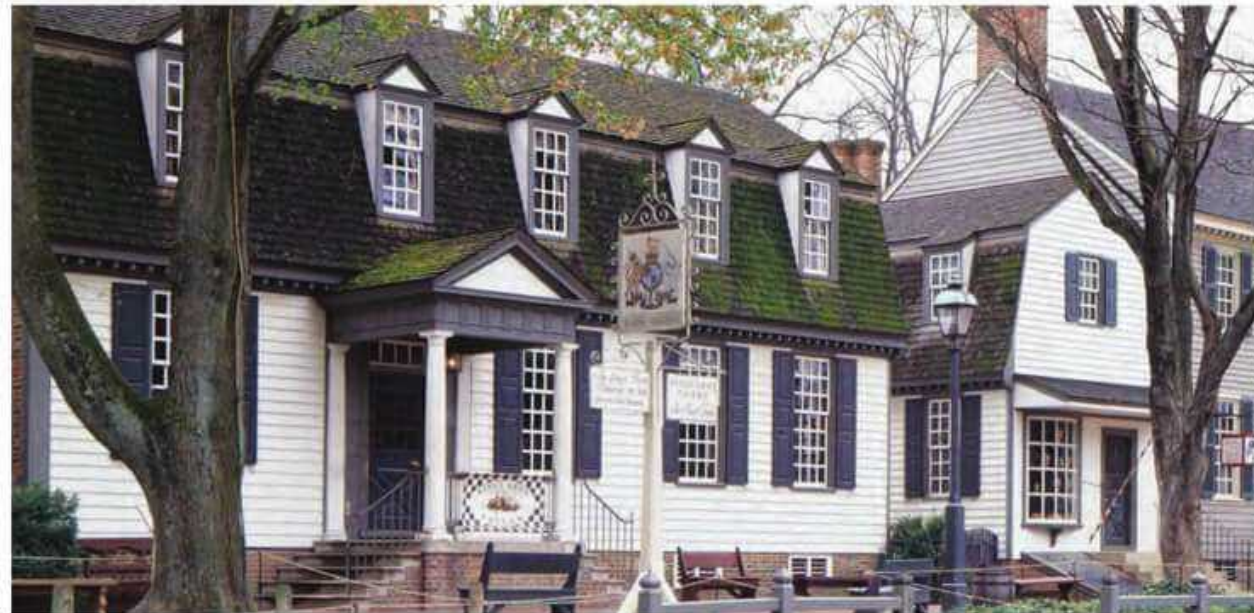
There are many buildings in Colonial Williamsburg using materials purchased from The Joinery Company.
